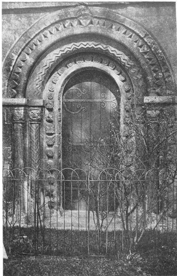
OLD NORMAN DOORWAY OF THE CHURCH AT IFFLEY, SHOWING THE FRANK AND SIMPLE DECORATIVE IDEAS OF THE PERIOD.
