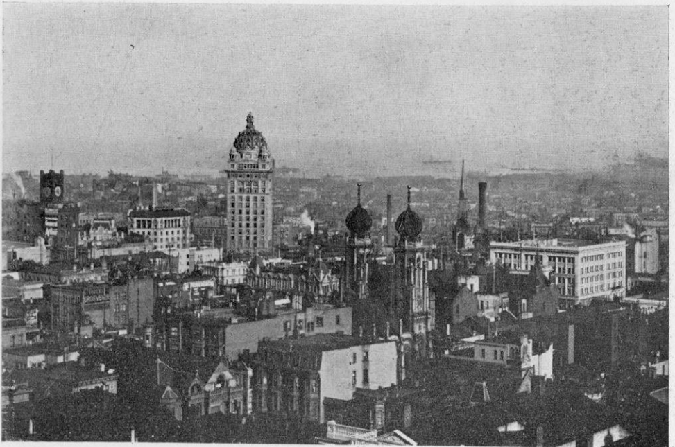
IN THE BUSINESS CENTER, SAN FRANCISCO
