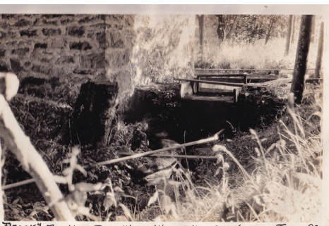
"SILVER BROOK" THE MAIN DAM WHEN WATER HAD CUT UNDER JULY-1931
