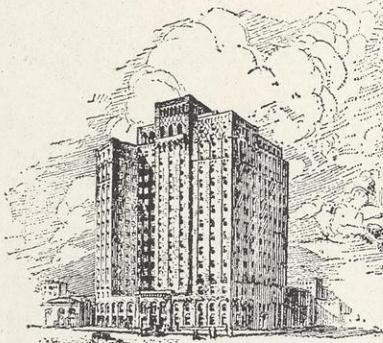
Chester Ave & East 13 th Street Cleveland (Under Construction)
