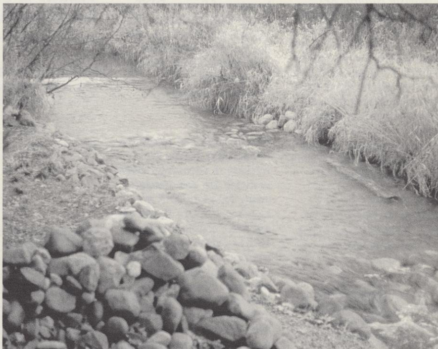
Rock sills on Chaffee Creek protect this spawning riffle.
