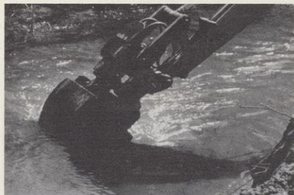
A backhoe scooping silt above a spawning bed. Photo courtesy of U.S. Forest Service
