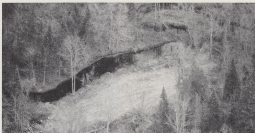
Foresters dug fancy ditches in trout streams to trap silt and sediment and they really work. Even this 150-foot-long, 20-foot-wide sand trap must be cleaned out annually.
