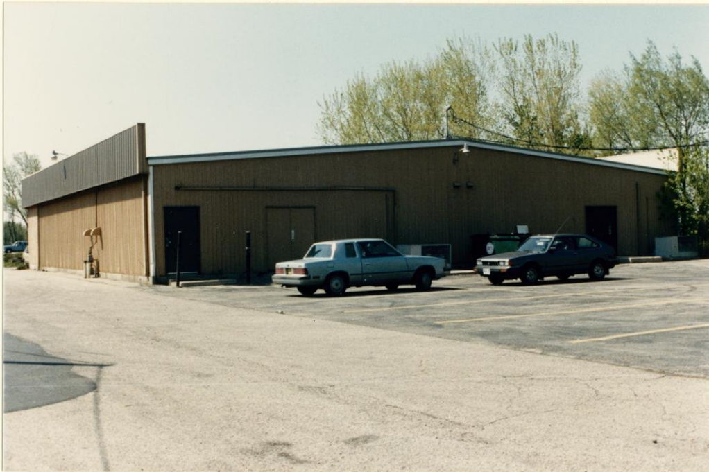
Back of building showing parking and rear entries. The double door has been sealed off as an entry.
