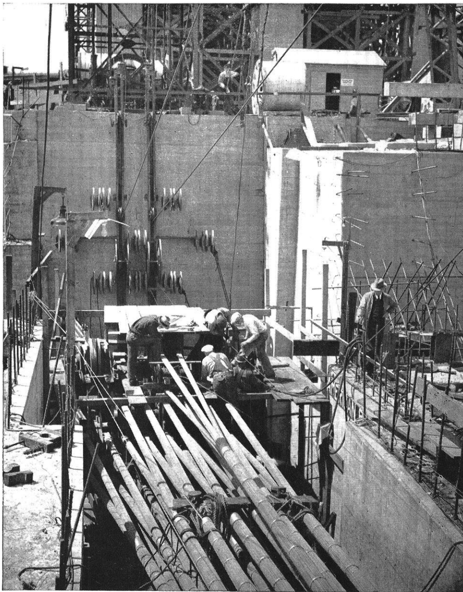
—General Electric Review Strands of cable in place at the San Francisco anchorage
