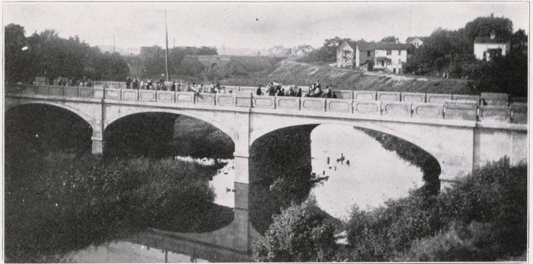
Middle Street Bridge.
