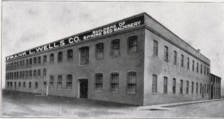
View of the Frank L. Wells Factory
