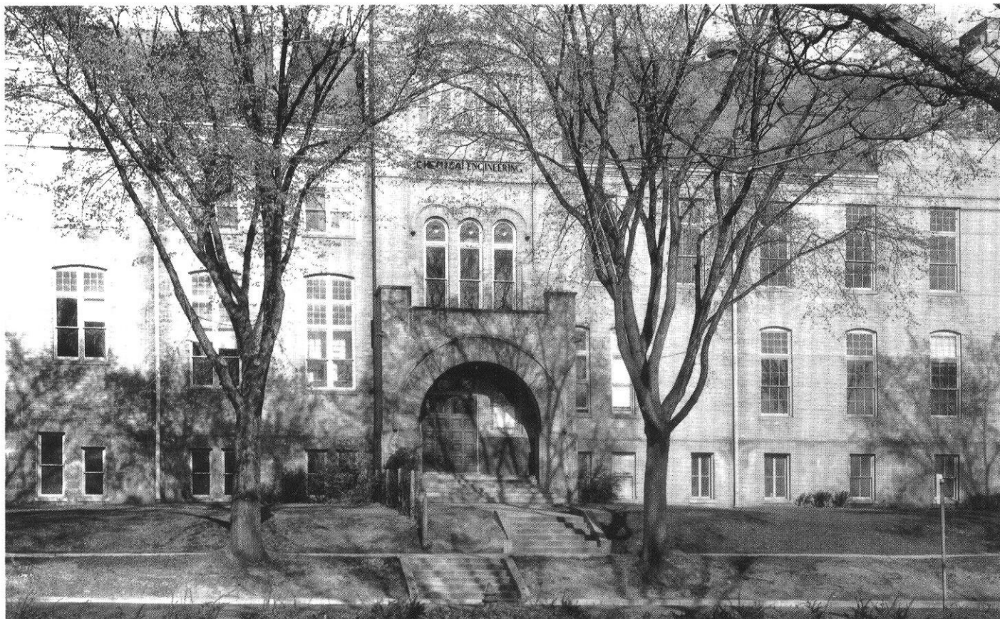
The Engineering Campus has experienced more than curricula changes through its years, as exhibited by this picture of the old Chemical Engineering Building.
