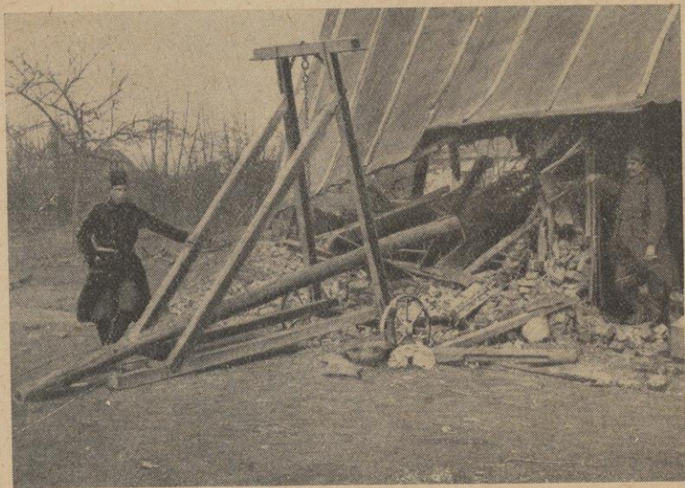
A battering ram used by the Germans for destroying houses before their retreat.
