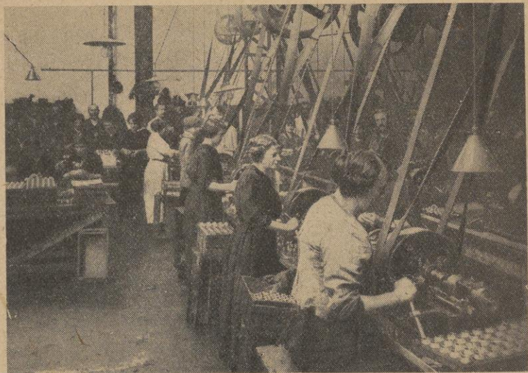
the Suresnes Electric Works. Manufacturing shells.
