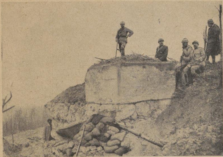
German pill-box captured near the Malmaison fort on the Chemin des Dames, 1917.
