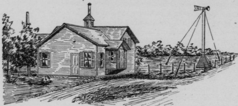
FIG. 5.—View of P. H. Kasper's cheese factory with funnel of sub-earth duct.
