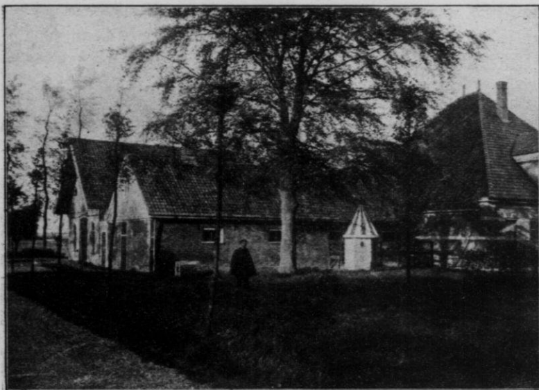
FIG. 25.—Farm buildings at De Ripp, North Holland. J. W. Decker in foreground.
