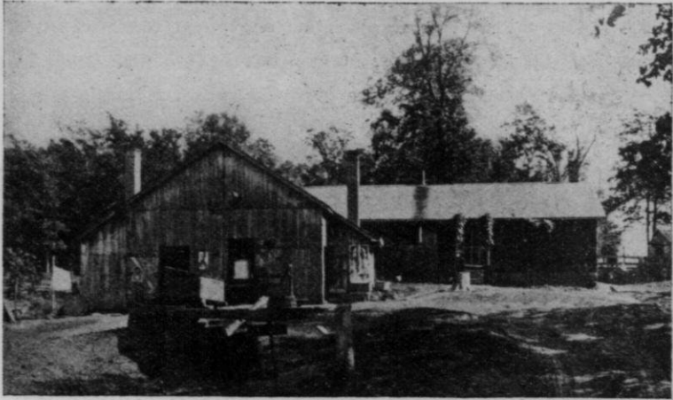
FIG. 2.—The Raub Factory, 3\frac{1}{2} miles east from Monroe, Wis. The cheesemaker, Mr. John Wyss, lives in the wing. The barrels in front are for the whey, each patron having a barrel. The trough over the barrels has a hole over each and the whey is thus distributed to the different barrels.
