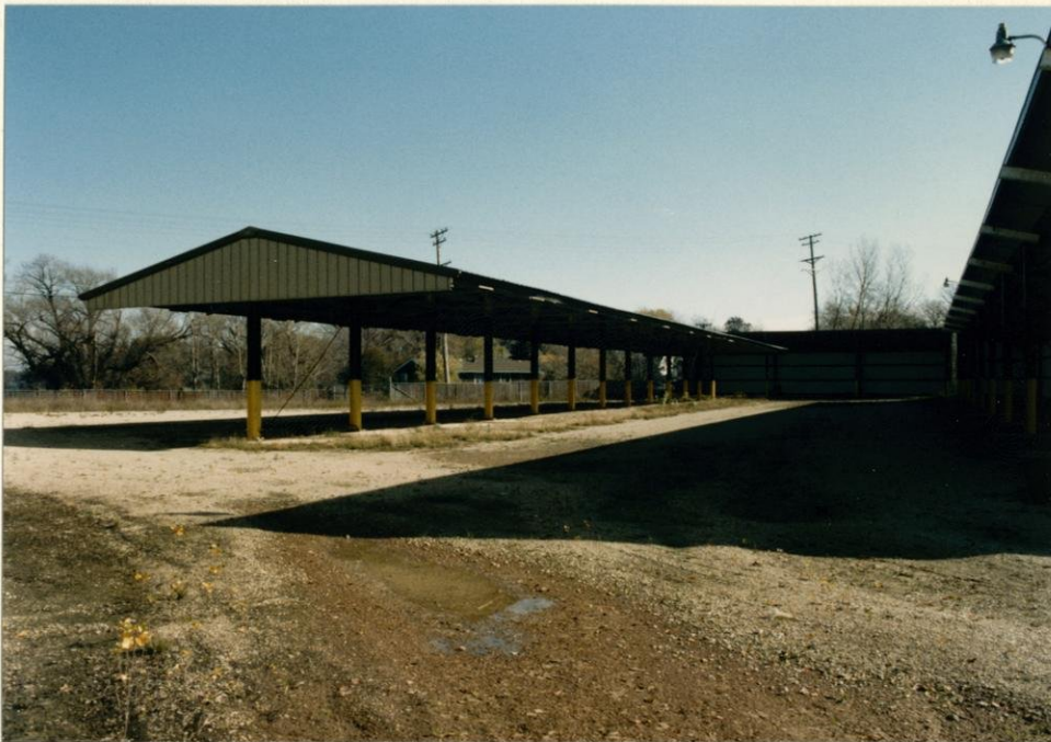
View of cantilevered roof storage area. Note chain link fence and wooded residential area in background.
