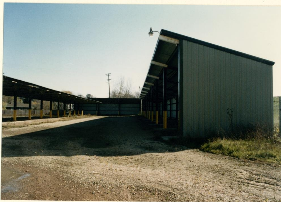
View of sheds and cantilevered roof storage area. Note compacted gravel driveways and evenly spaced concrete footings.
