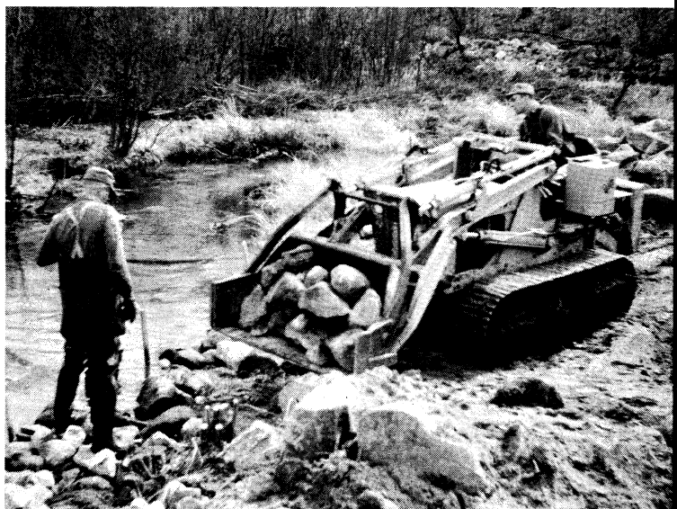
. . . was narrowed and deepened with wing-deflectors and bank covers. Note the dark protective pool in the bend at the left (below).
