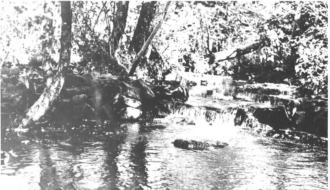
Another form of low dam which is desirable because of its natural appearance. It is made from rocks available at the stream site, and is an imitation of the natural stair-step pattern of very steep stream beds. (Minn. Dept. of Conservation)
