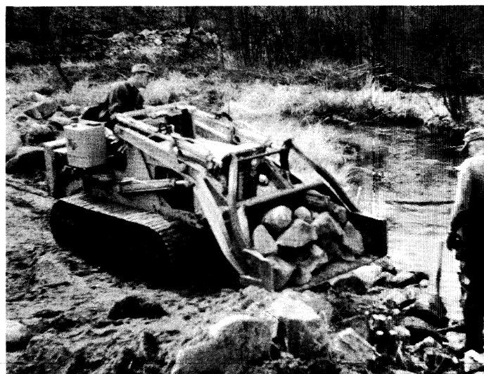
4-5 Revetting with rock behind the overhang and covering with rock.
