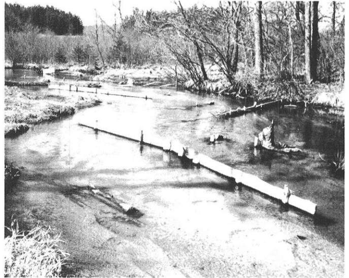
Flimsy construction does not pay ten years later. Simply deflecting the current with plank wings wasn't enough. The bank has been eroded back several feet and winter ice formations have lifted the structures (see especially the plank in the background). Now most of the current goes under or around the structures and the stream remains wide and shallow.
