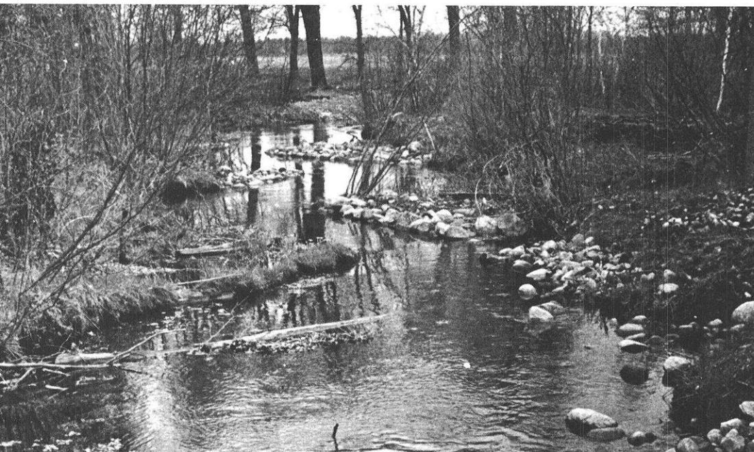
Wing-deflectors in a stream, showing alternating pattern.
