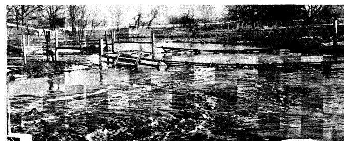
Floodgates performing during a flood.
