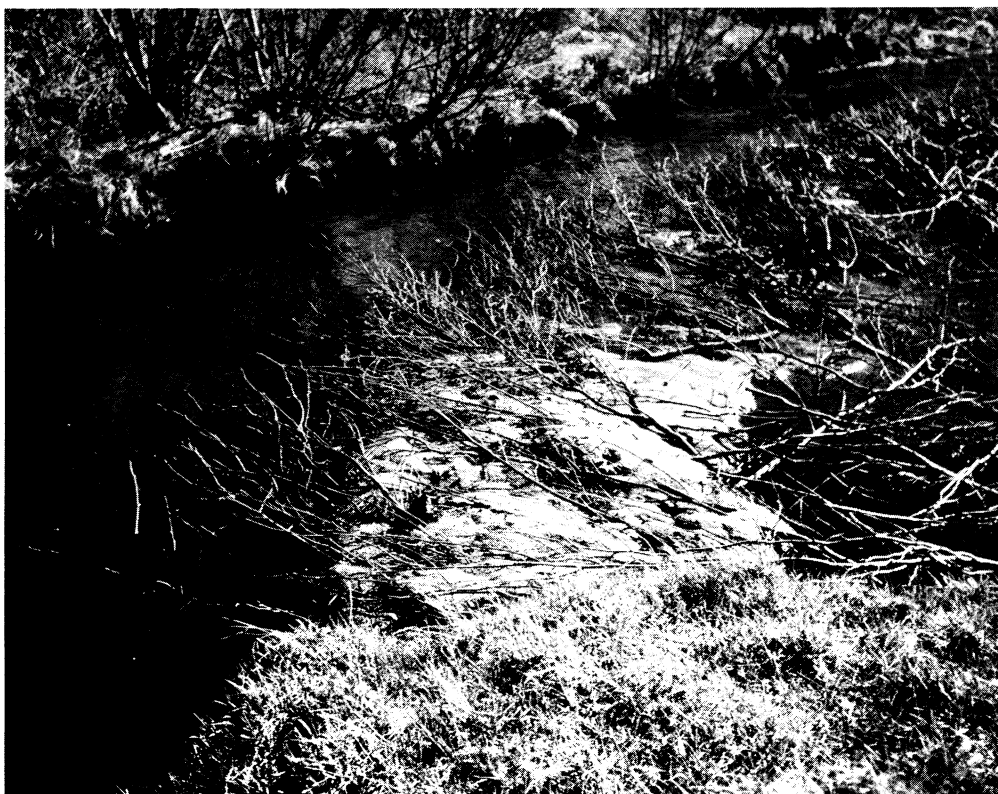
Silt and sand collect at a point bar extension of a wing-deflector. The view here looks downstream from one deflector. Brush is placed along the convex bank at this point to help tie down the fine sediments. Grass will soon cover the bar and make it a permanent part of the stream bank.
