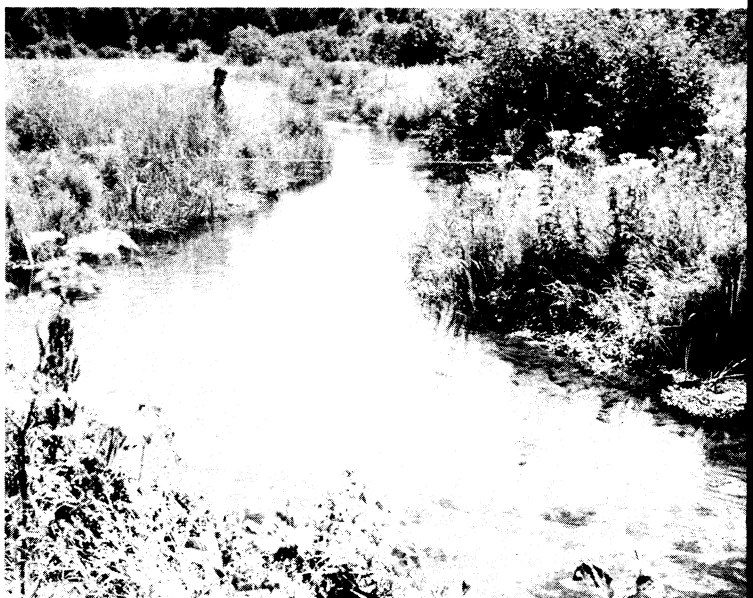
. . . was narrowed and deepened with wing-deflectors and bank covers. Note the dark protective pool in the bend at the left (below).
