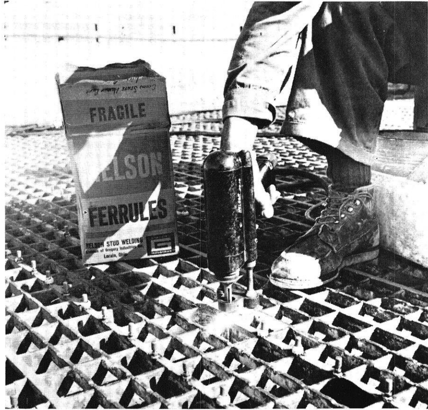
Photo shows a closeup of non-skid studs being welded in place.
