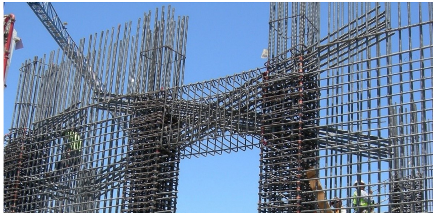
Figure 2.8: Coupling Beam Under Construction (Courtesy of R. Lequesne).
