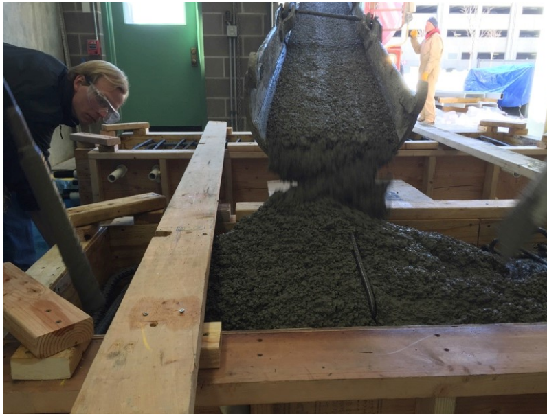
Figure 3.10: Casting of End Blocks.
