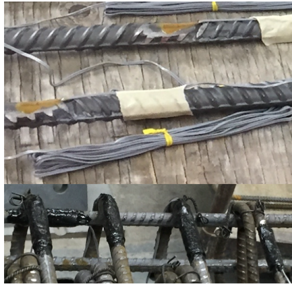
Figure 3.16: Strain Gauge Installation (Top) and Strain Gauges with Finished Coating (Bottom).
