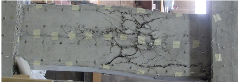
Figure 4.1: Shear Failure of Specimen CB1.
