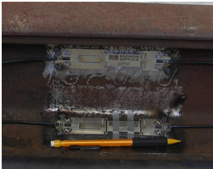
Figure 4.7 FO sensors locations on the rail
