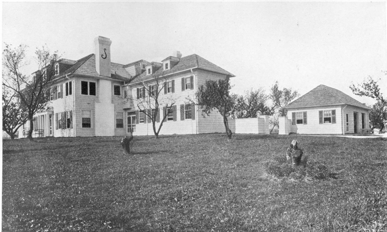
The exterior of George K. Smith's country house near St. Louis, showing the convenient relation of garage to the house and the high wall that conceals the kitchen garden from a too familiar view.
