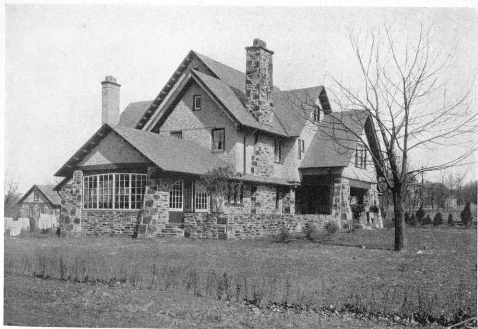
A MODERN STONE AND CEMENT HOUSE: BUILT IN MERION, PA.: DAVID KNICKERBACKER BOYD, ARCH- ITECT.
