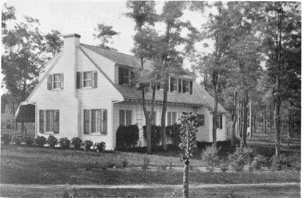
TWO VIEWS OF A MODERN COLONIAL HOME BUILT FOR G. E. FAHY, LOCUST VALLEY, SHOWING RIGHT PROPORTION AND EXQUISITE SIMPLICITY: JAMES W. O'CONNOR, ARCHITECT.
