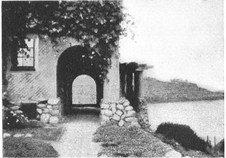
AN ARCHED PASSAGEWAY IN THE NORTHERN FAÇADE.
