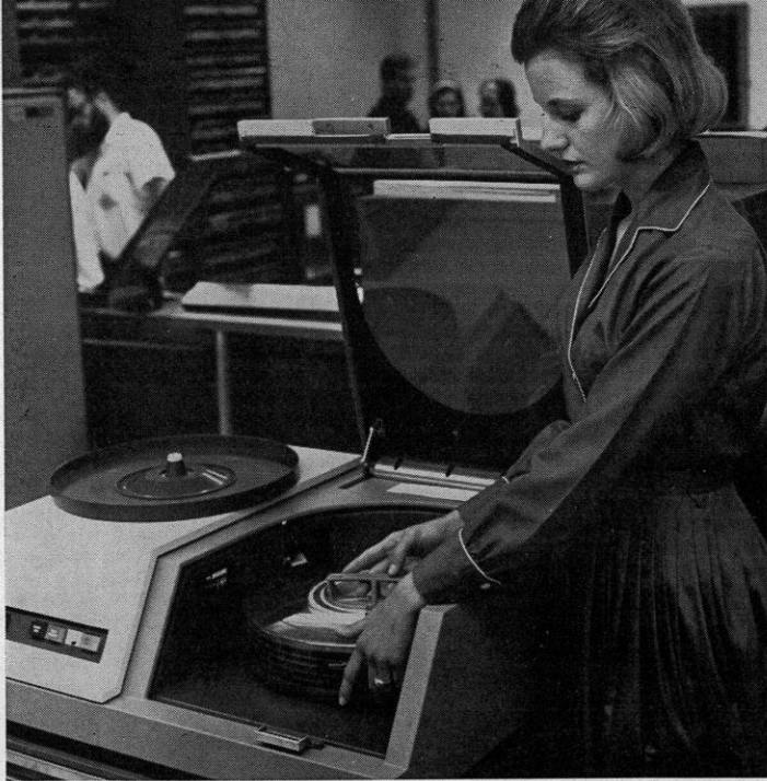
Sandy Lee demonstrates the disc-pack unit of the new 1460 computer.
