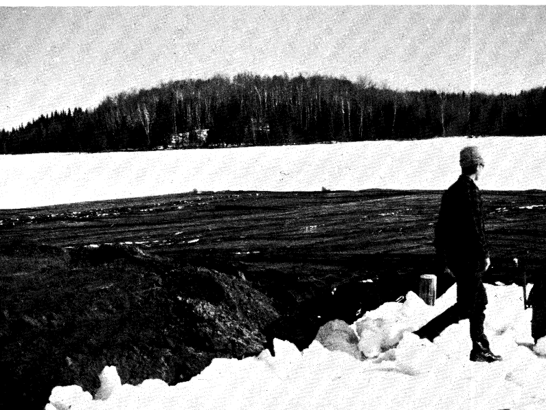
Sand blanket laid over plastic on the ice.
