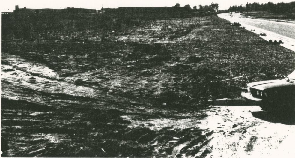
Fig. 4i Looking west along Royal Avenue across subject's retail service area.
