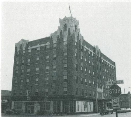
327 (15 S. High Street) Monterey Hotel 1930 Paul Frederick Olsen, architect (firm of Frank Perry, Chicago)
