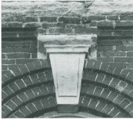
11 Otto F. Meyer Building 1865-70
