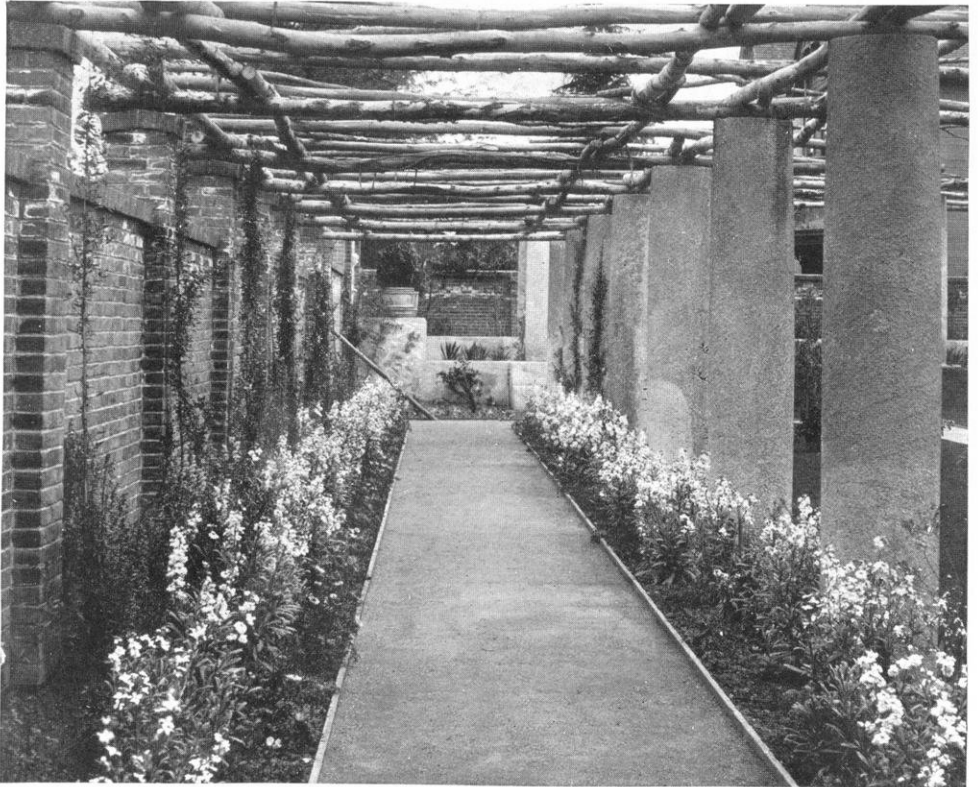
TWO VIEWS OF WESTERN PERGOLA CIRCLING A BRICK WALL, GIVING THE EFFECT OF THE USE OF THREE KINDS OF MATERIALS, CONCRETE, BRICK AND RUSTIC: A CHARMING METHOD OF COVERING A GARDEN PATH.
