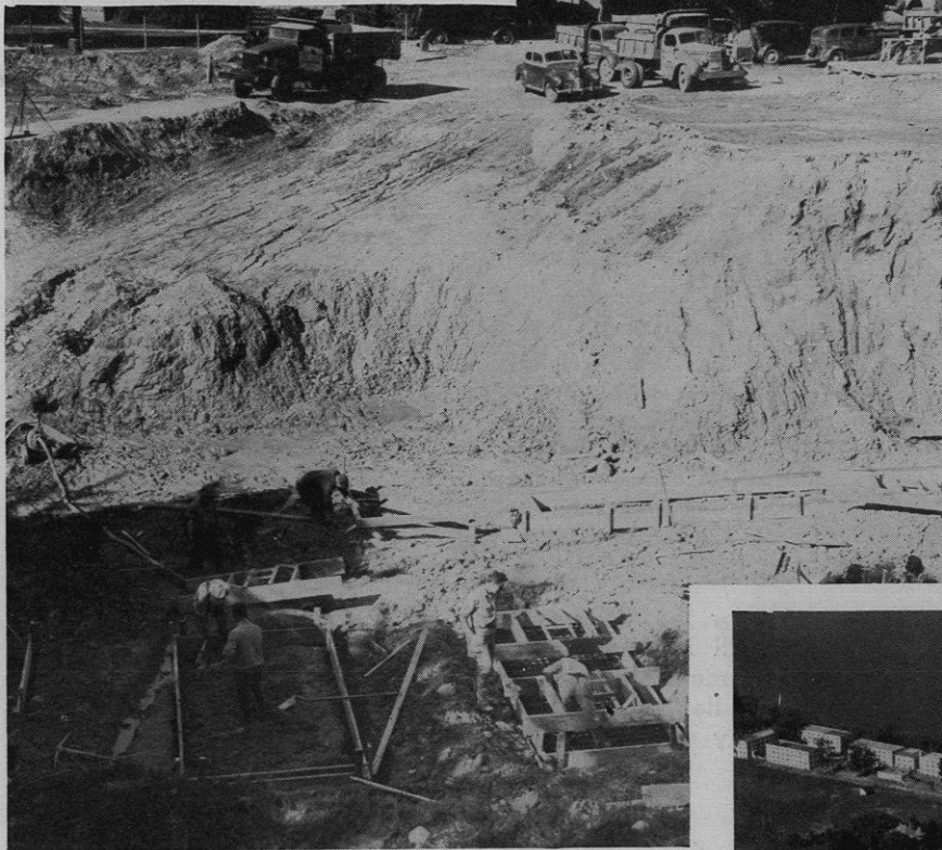
WORKMEN ARE SHOWN laying the footings for the University's new $300,000 men's dormitory. The building is to be ready for use by Sept., 1947, will cost twice as much per occupant as did pre-war construction.
