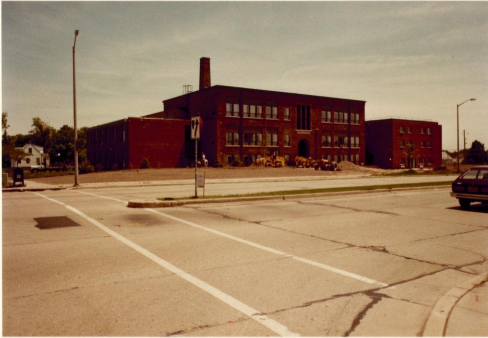
Front view of 56 elderly apartment units. The middle part is the original school structure, built in 1931; the left wing was added in 1952; the right 3-story addition was built in 1981-82.
