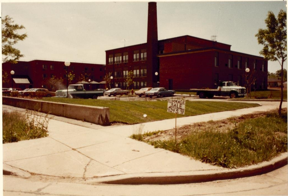
Back view showing parking.
