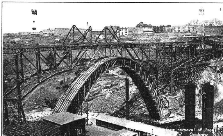
FIG. 2.—South 120 Foot Arch with Centers Struck.
