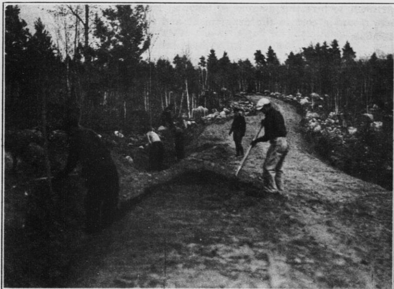
Truck trail construction under ECW program.
