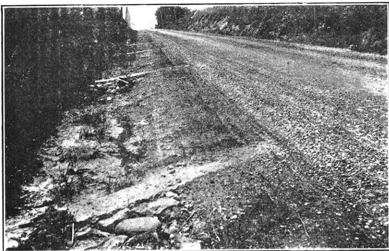
Concrete "breakers" as used on Maryland roads. A simple device to prevent washing of shoulders and gutters.
