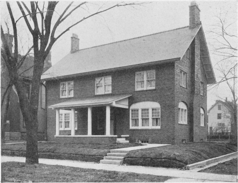
SOUTH FRONT OF CRAFTSMAN HOUSE BUILT BY G. C. KINSMAN, DECATUR, ILL.
