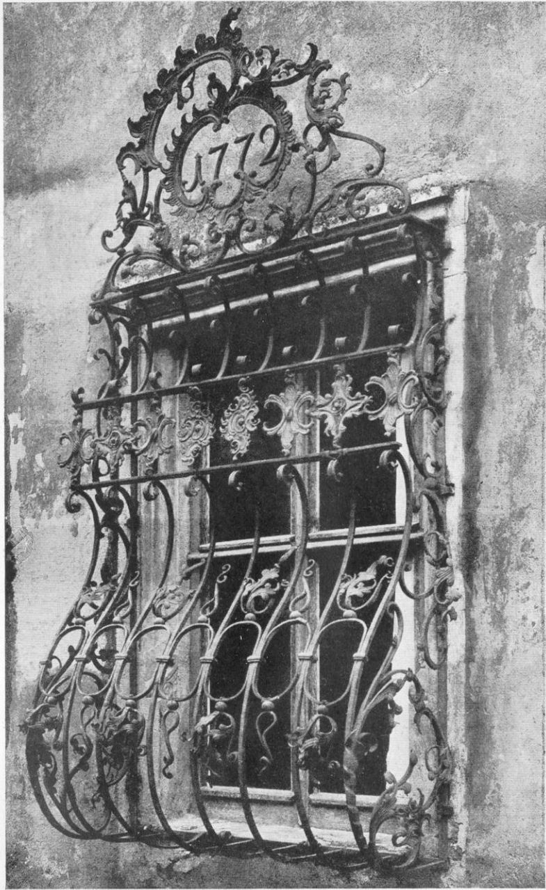
WROUGHT-IRON GRATING TO PROTECT WINDOW OF ANCIENT HOUSE
