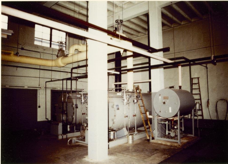
Interior of boiler plant: Kewanee boilers
