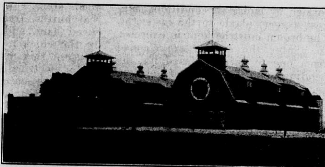
The Barns on a modern dairy farm
