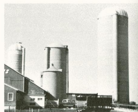
Alan Barta farm, Two Creeks. A contrast of sizes and ages of concrete silos. Bunk feeder attached to the large silo on the right. Note almost flat roof on the medium silo in center.
