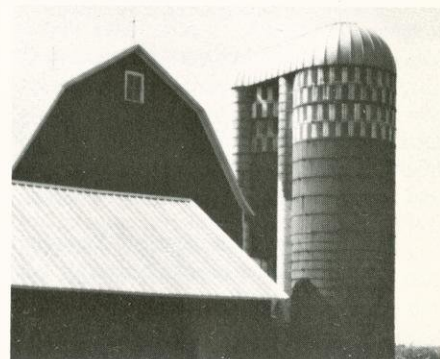
Example of twin silos with a common roof and top unloader. When one silo is empty, the unloader is raised and transferred into the other silo. Concrete stave type built in the late 1950's. Harvey Guse farm, west of Maribel.
