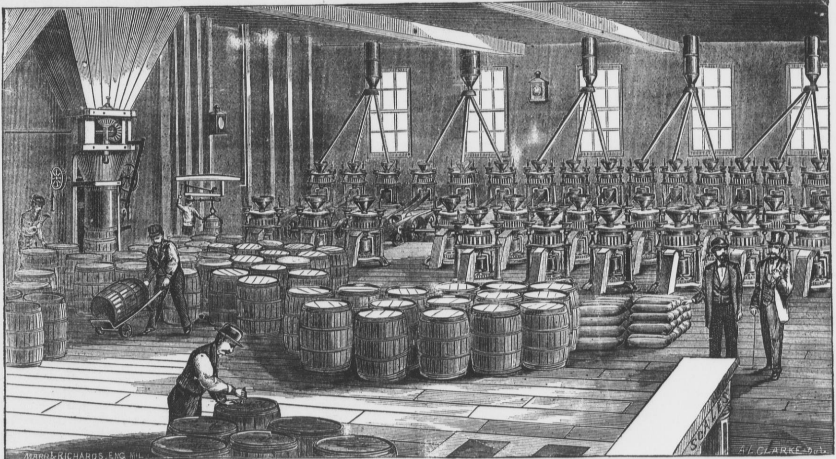
FIG. 2. INTERIOR VIEW OF THE GRINDING FLOOR OF THE MILWAUKEE MILLING CO.'S NEW MILL, MILWAUKEE, WIS.
