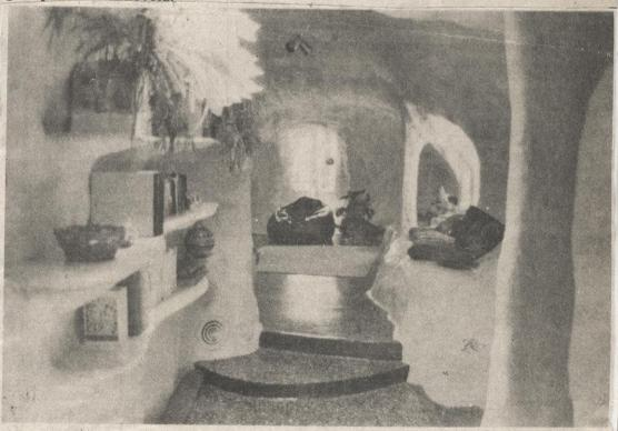
The floors, walls and ceilings all blend together in the Habitable Sculpture to give a maze effect to the main floor of the structure. The interior, like the exterior, was constructed by spraying polyurethane foam onto a polyethylene air structure.
