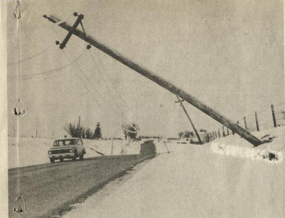
All the old poles broke and the new ones barely stood the strain during recent ice storms. Power and telephone poles along a five mile on Highway 80, south of Highland, were wiped out. Over 80 power poles needed replacement and at least that many telephone poles. Note the new telephone poles going up along the left side of the road.
