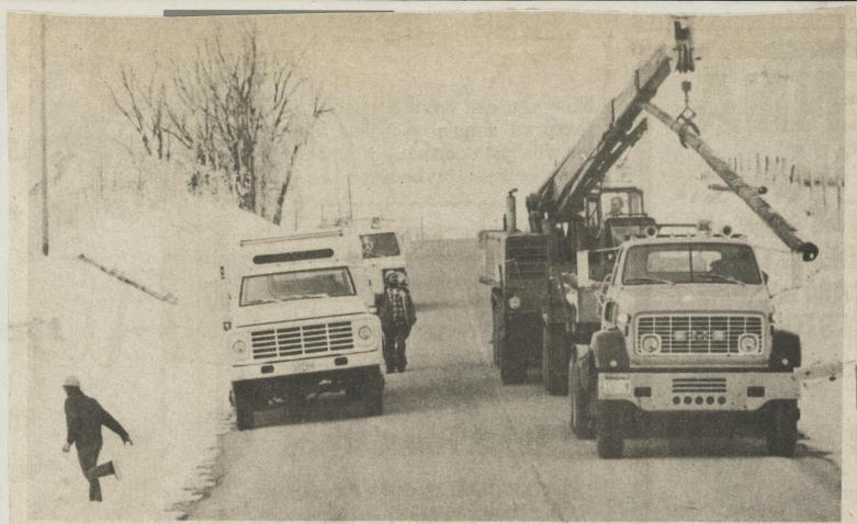
Heavy equipment and a lot of man hours are required to repair damage received from the recent storms. Above an electric company crew unloads poles as the telephone men repair lines.
