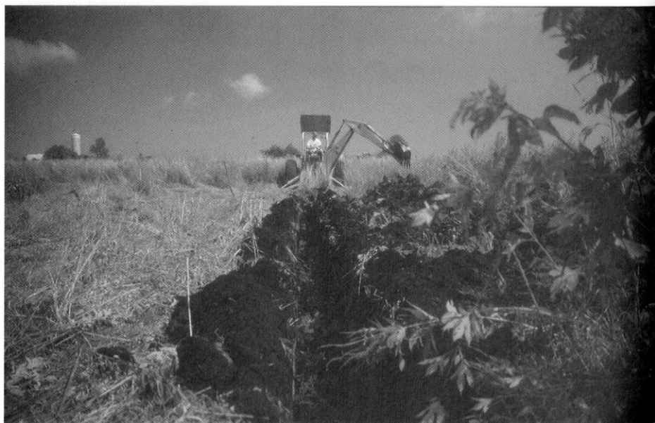
Figure 3: Search and destroy mission on a backhoe. Finding tile lines was tedious work. Trenching across entire waterways, to a depth of 6', usually revealed buried tile lines.
