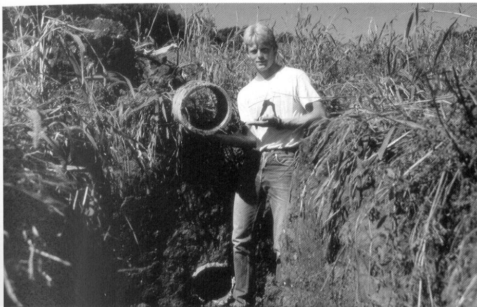
Figure 1: Subsurface tile lines were 4–9' below ground. Average diameter was 4–6". Pictured here is a portion of 12" tile held by Kyle Drake.
