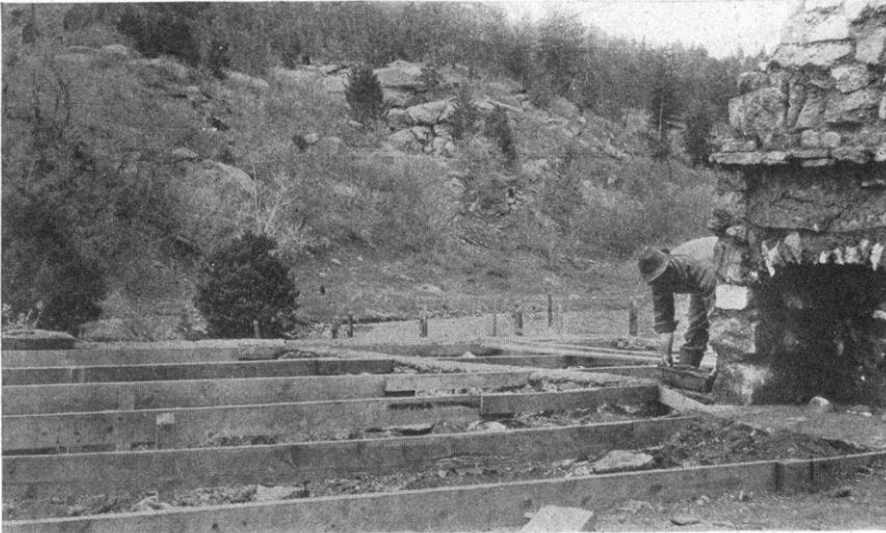
THE LONE WORKMAN PUSHED AND ROLLED HUGE ROCKS FROM THE HILLSIDE TO FORM A CAVERNOUS SIX-FOOT FIREPLACE.
