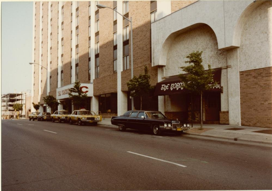
Dayton Street main entrance and Normandy Restaurant entrance
