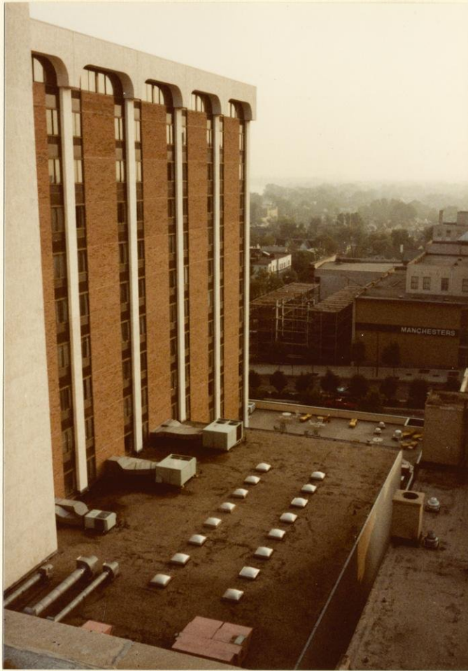
Guest Room Tower, pool and banquet room. Roof and patio deck
