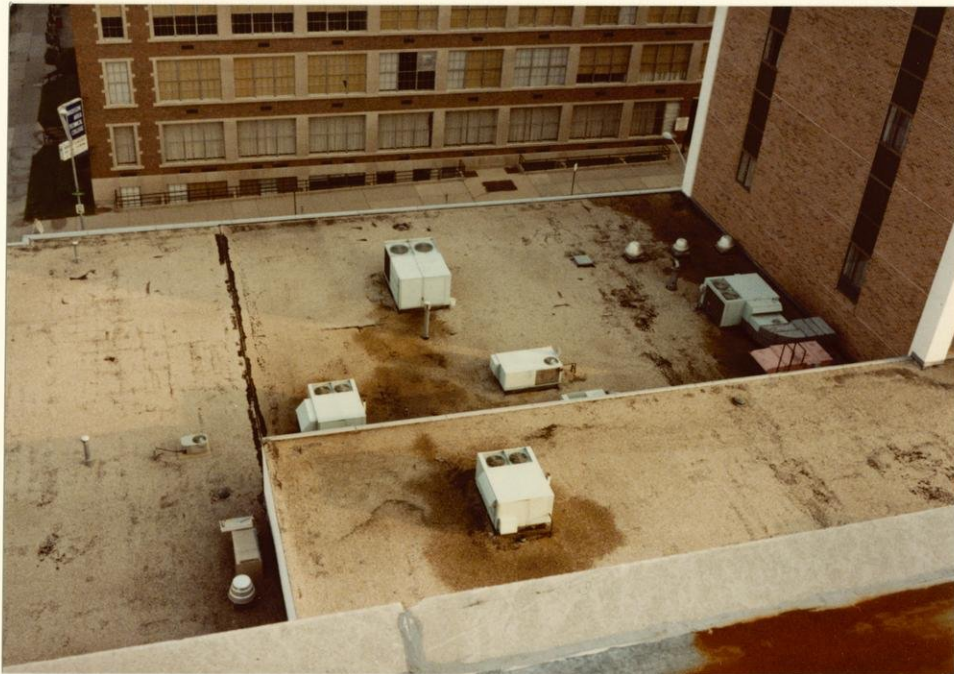
Area of roof on which proposed addition is to be built
