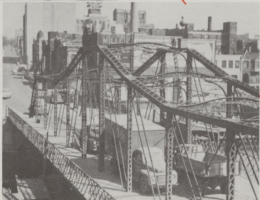
→ A new $1,100,000 double span bascule bridge will soon replace this outmoded Juneau Ave. swing bridge.
