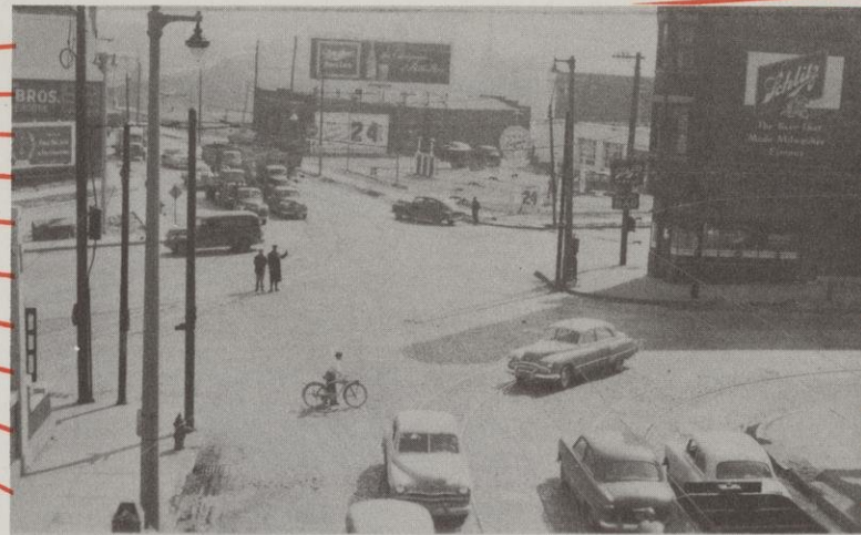
▲ A proposal to build either a W. St. Paul Ave. or W. Clybourn St. underpass in 1952 at this N. 6th St. intersection is receiving serious study.
