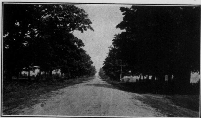
Nine-foot Gravel Road, town of Summit, Waukesha County, built in 1914 at a cost of $2,200 per mile, including grading and culverts.
