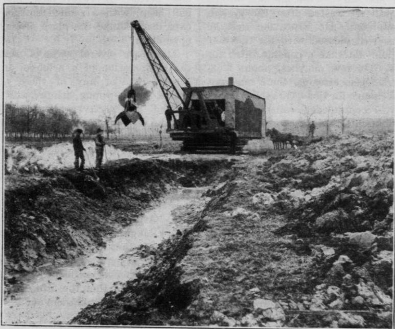
Figure 9. An Open Ditch with Dredge.
