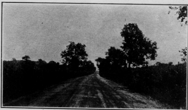
Nine-foot Gravel Road, town of Delafield, Waukesha County, built in 1913, at a cost of $1,800 per mile, including grading and culverts, and surface treated in 1915.
