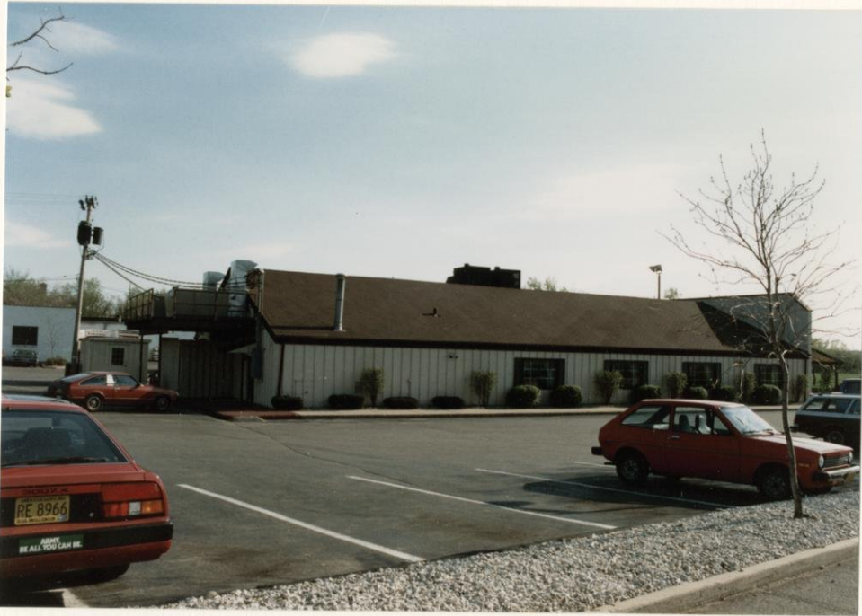
Looking at north side of Ponderosa building from north property line. Note HVAC equipment on extended platform at rear of Ponderosa.
