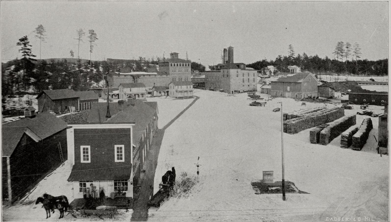
BIRDSEYE VIEW OF LEININKUGEL BREWING CO.'S PLANT.
