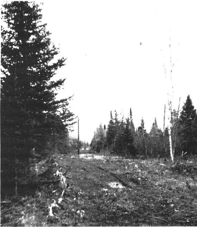
Each antenna leg courses through the woods along thirty foot right of ways. If Phase II is implemented, the wires will be buried.
