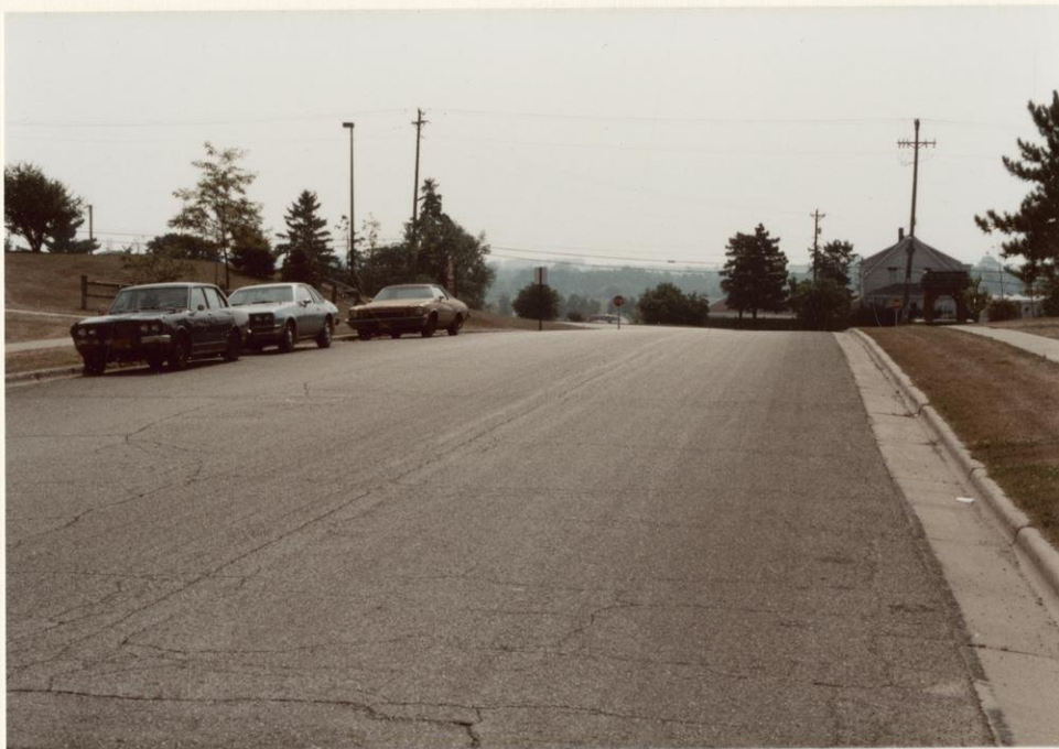
Looking east along Traceway Drive toward Fish Hatchery Road
