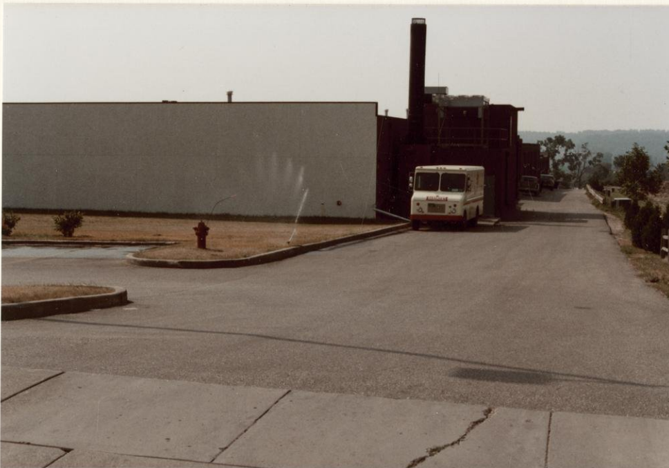
Looking south, view of service drive from Post Road
