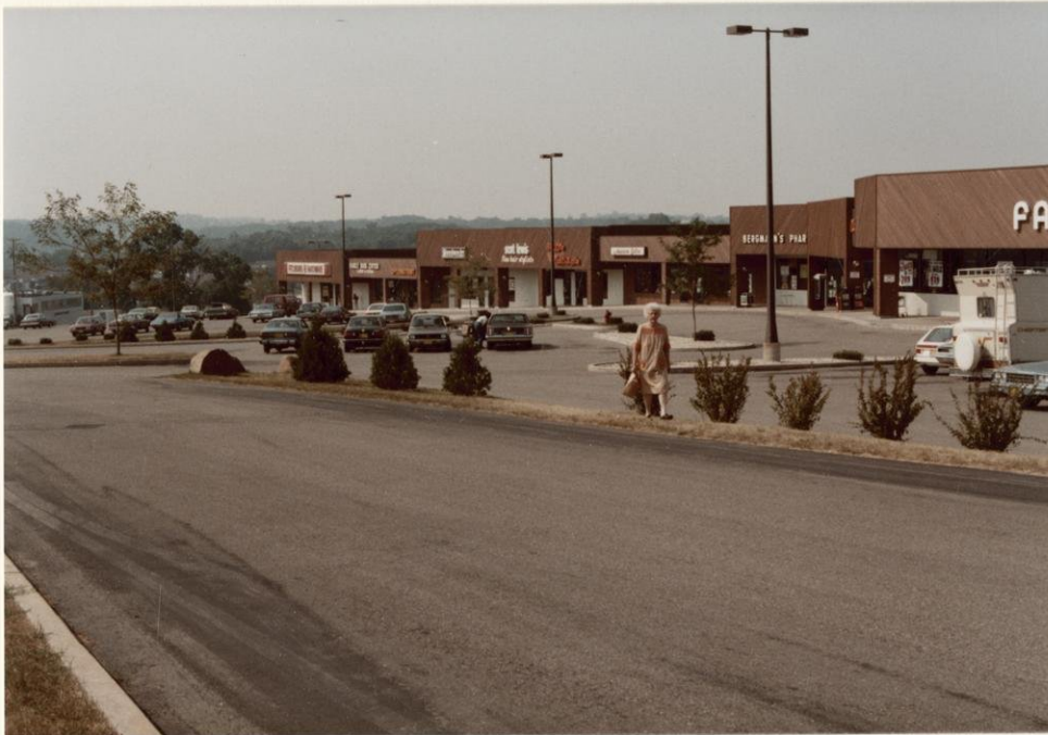
Front view of the center looking southwesterly
