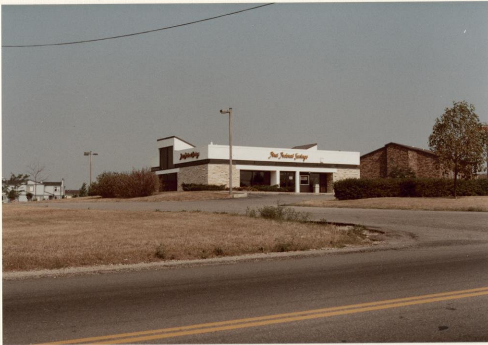
View showing outlot and its entrance drive at north end of the site
