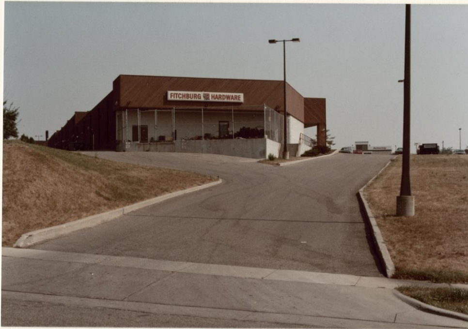
Traceway Drive entry at southern end of center
