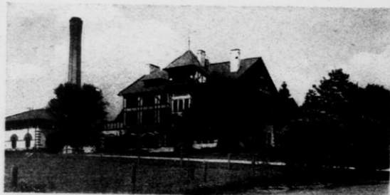
The Dairy Building
