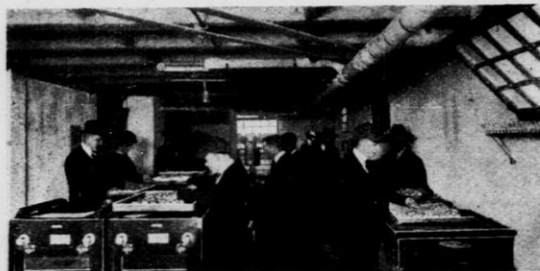
Incubator Room at Poultry Building
