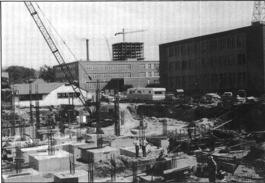
The foundation of the Engineering Research Building, 1967.
