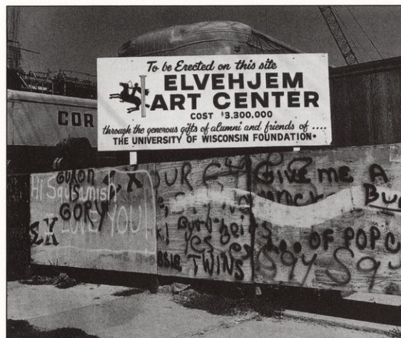
Figure. 2. A portion of the infamous fence around the construction site.
