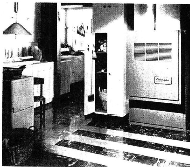
Fig. 5.—This is the Carrier Weathermaker, a combination heating and air conditioning unit, here installed in a utility room. In this plan, air conditioner, laundry facilities, and kitchen are grouped in one area, or "core unit", thus reducing heavy wiring and plumbing expense.
