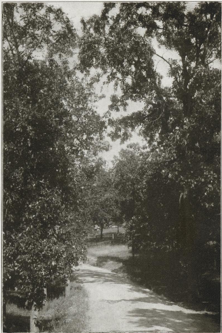
LAKE MENDOTA DRIVE. RELOCATION ON WARNER FARM
