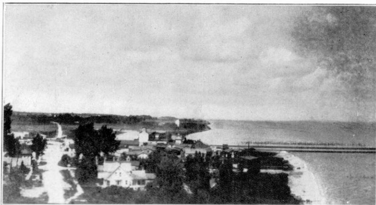
Fig. 1. View northward at Kewaunee, showing the accumulation of shore drift on the south side of the pier.
